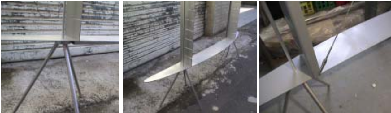
Above: Detail of the acrylic partition screen leg system, detail of the fitted cross brace to the back of the partition
