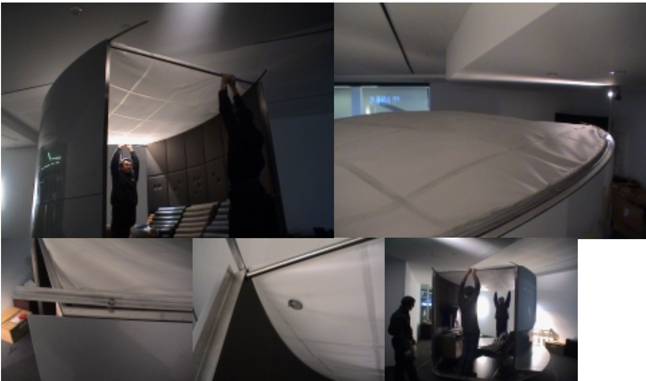
Above: Images of the prototype inflatable ceiling fitted the Screen Lounge pod 01 including the rope track temporary mounting.
