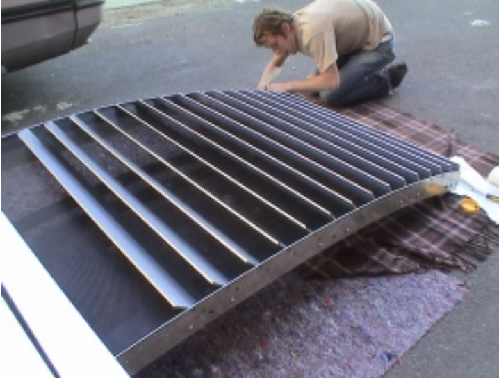
Individual louvres are screwed into the support frame of the louvre wall. The central membrane of black metal mesh can be seen behind the louvres
