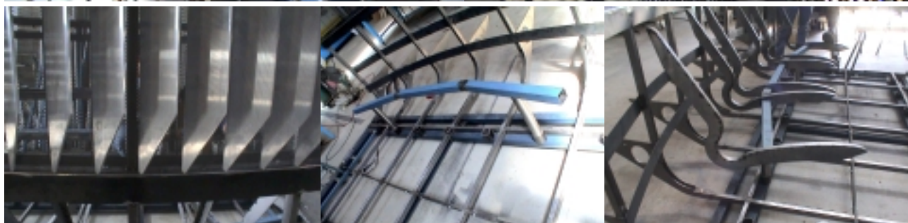
Clockwise from top left: Louvre array in place on the first production Screen Lounge pod, detail of the reflective inner surface of the louvre array showing the functioning of the discontinuous and fragmented porous surface as proposed in report 17, detail of the fixing of the louvre array to the steel skeleton, detail of the seating beam and it's floor fixing system, detail of the seating support frame, view of the complete frame.
